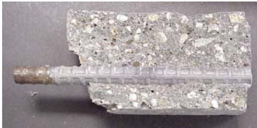
Figure 8. This photo shows the treated rebar still embedded in the concrete and the portion of the rebar that was exposed to the corrosive environment.
