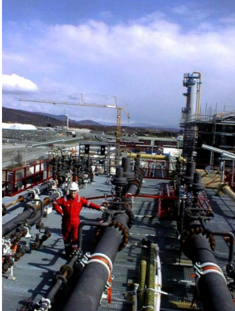
Figure 5 Ü Onshore Pipeline Installation
